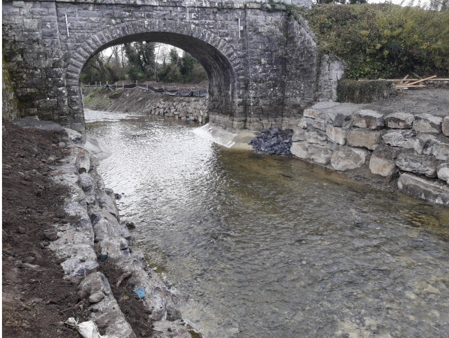
Figure 10: UB154 Railway Bridge
