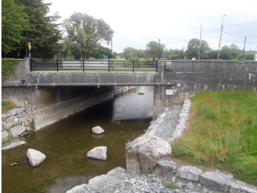
Figure 8: Regrading of Dunkellin complete
