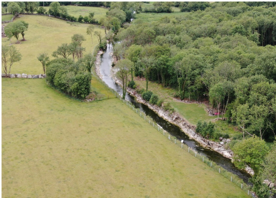
Figure 7: Reinstated Section of Dunkellin in June 2020, following Regrading Works
