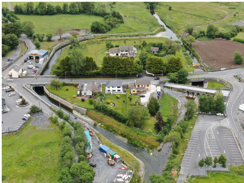
Figure 1: Completed Craughwell Village Bypass and River Deepening Works
