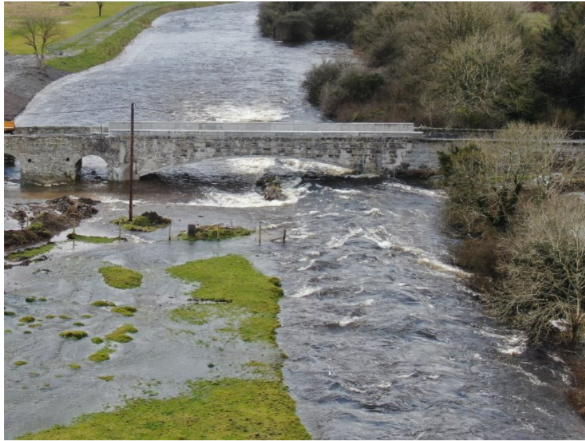
Figure 4: Flood Waters at New Dunkellin Bridge February 2020
