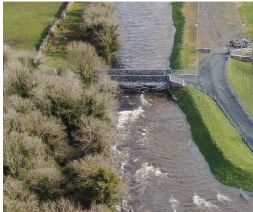
Figure 5: Flows through new bridge at Killeely Beg February 2020
