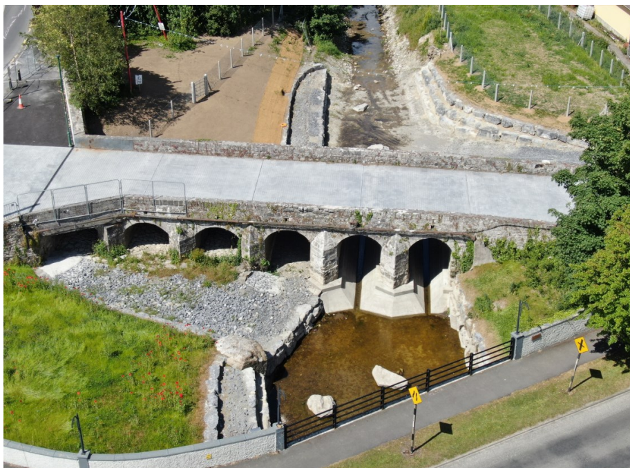
Figure 9: Deepening of Multi-arched bridge in Craughwell complete
