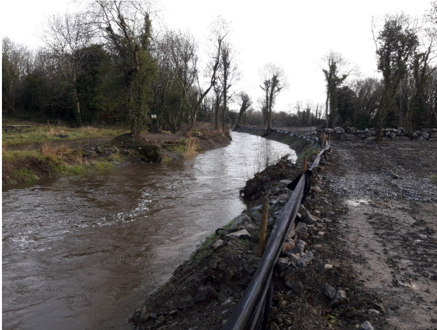
Figure 6: Regrading of Dunkellin during Construction in 2019
